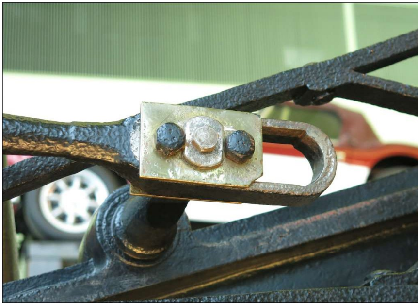
Figure 33. PS Industry Riverside Museum, Glasgow. This detail shows the sliding joint, part of the Watt equivalent straight-line mechanism used to keep the steam cylinder crosshead and piston rod in alignment with the cylinder.
