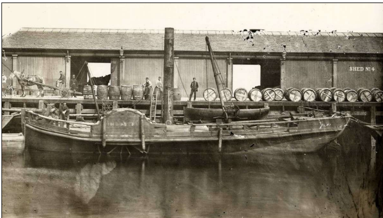
Figure 1. The Paddle Steamer Industry transported cargo between Glasgow's docks and the deep-water port at Greenock. Seen here berthed alongside the East India Harbour, Greenock around the 1850's (5) . The angle between paddles (floats) is 36 degrees confirming that the wheel has 10 paddles. ©CSG CIC Glasgow Museums and Libraries Collection.
