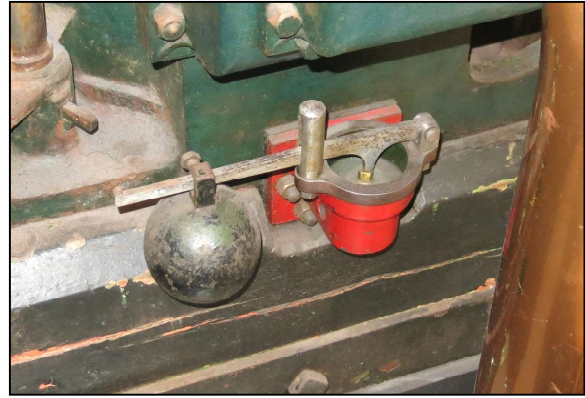
Fig. 27b. Safety valve on bottom of cylinder.
